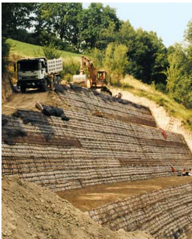
Tenax Rivel system for landslide repair.
