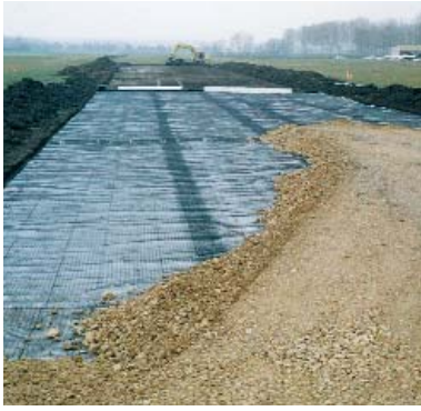
Soft soil stabilisation and separation using Tenax GT.
