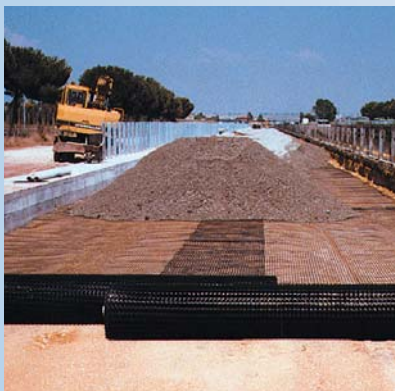
Low bearing capacity subgrade reinforcement with Tenax LBO geogrids.
