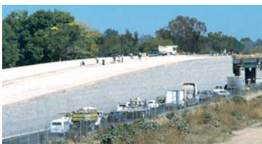
Bridge abutment with Tenax TT samp and concrete blocks.
