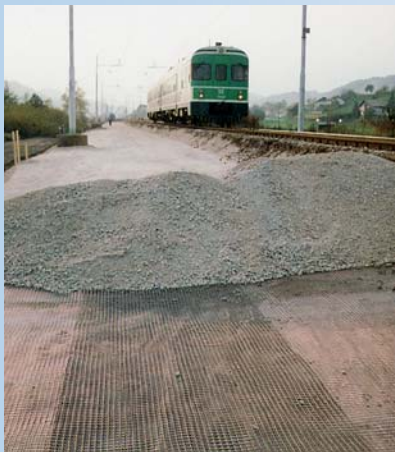
Railroad ballast reinforcement with Tenax LBO geogrids
