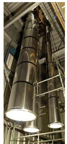
Internal view of different diameter tubular rooflights under test
